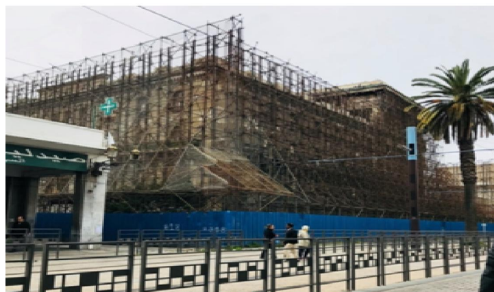
Figure 2: Image Showing the Lincoln Hotel in Casablanca, Morocco, Behind a Facade of Posts to Support the Last Walls Still Standing, Photo Karima Berdouz 2018.
