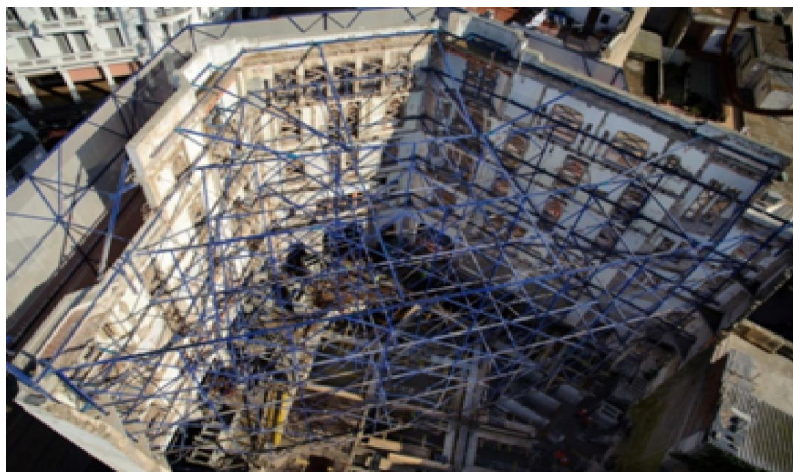
Figure 7 : Image Illustrating the Two Supported Facades Facing the Rue De La Banque De La Société Générale in Casablanca, Morocco.
